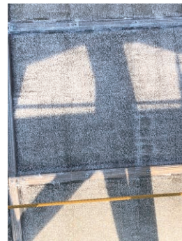
▲塗料半乾き状態
